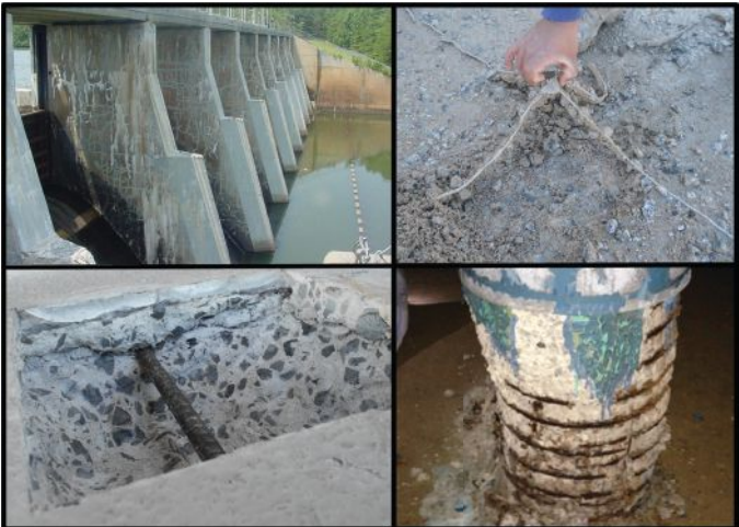
Fig. 2: Examples of materials-related distress top left to right: alkali-silica reactivity (ASR) and freezing and thawing damage (F-T); bottom left to right: corrosion, and chemical attack / corrosion
